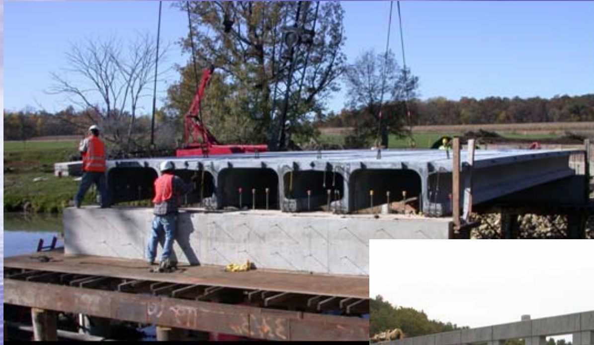
VDOT BT45 – no shear stirrups Rt. 624 Cat Point Bridge (FHWA 9 th -span) Richmond County, Virginia
